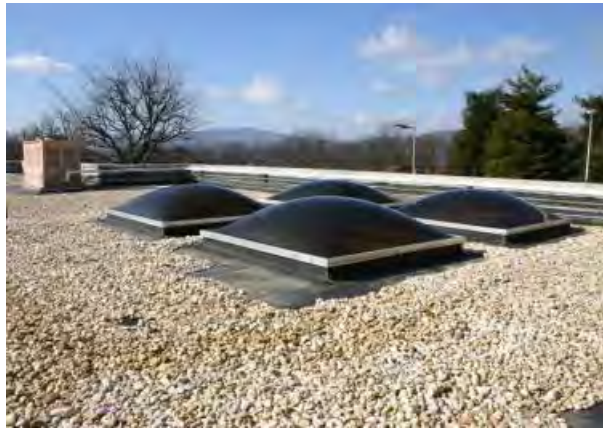
Ballasted roof over Emergency Department / Intensive Care Unit
