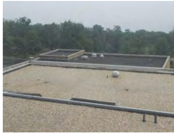
Ballasted roof over Emergency Department / Intensive Care Unit
