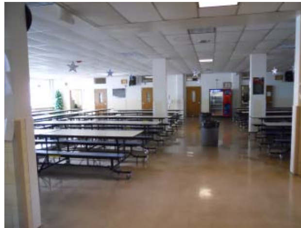
Photo 20 BMS – Vinyl Asbestos Tile
