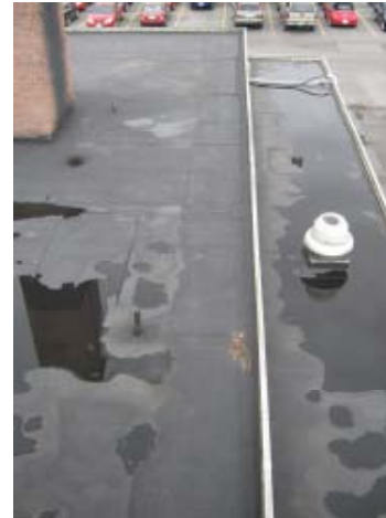
Photo 3 WMS - Roof-condition fair with ponding
