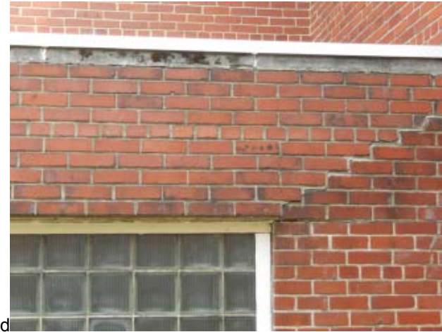
Photo 31 AHS - masonry cracking from settlement.
