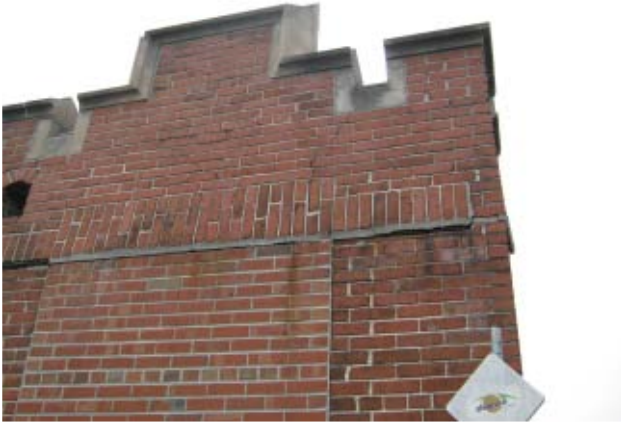
Photo 29 – AHS masonry needs repair / repointing.
