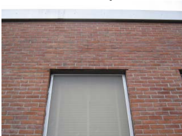
Photo 6 WMS - Exterior windows single glazed – rusting lintels
