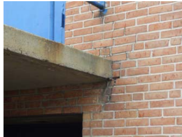
Photo 32 AHS - Damaged masonry at canopy.
