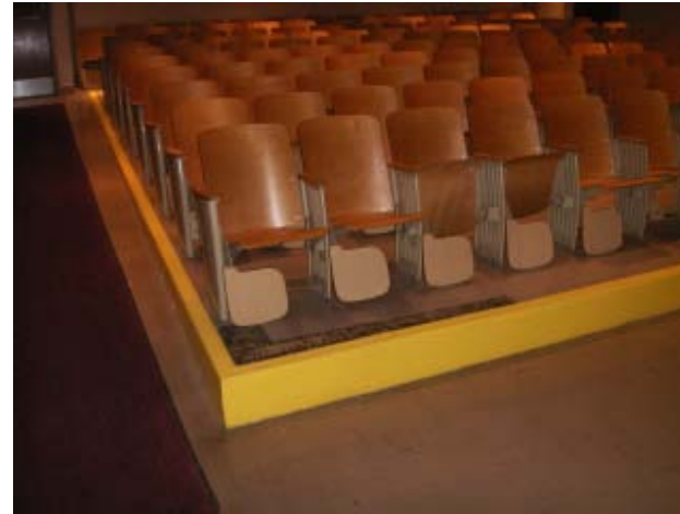
Photo 7 WMS – Vinyl Asbestos Tile
