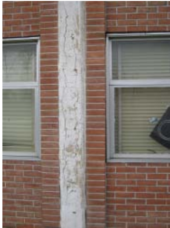
Photo 5 WMS - Column cracking
