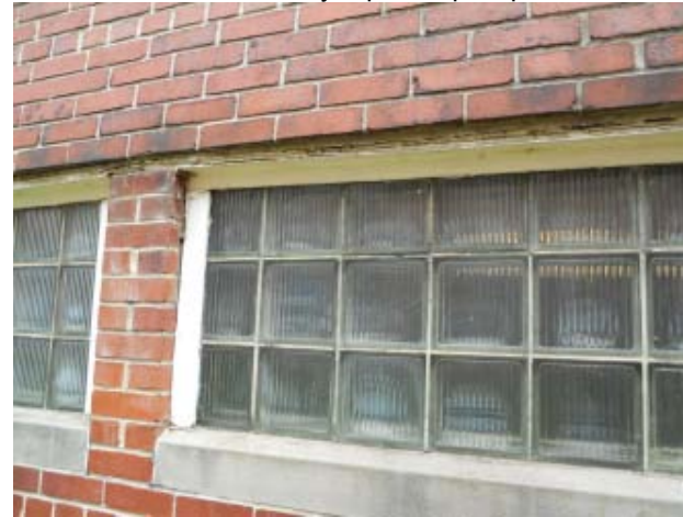
Photo 35 AHS - Exterior rusting lintels
