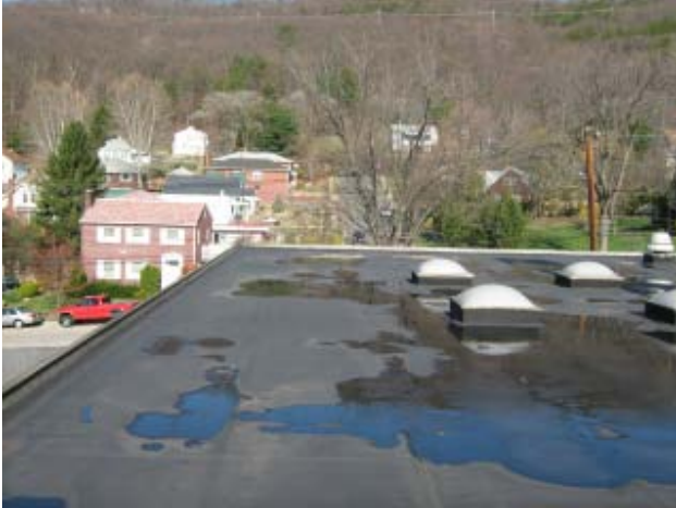
Photo 17 BMS - Roof, fair condition with ponding
