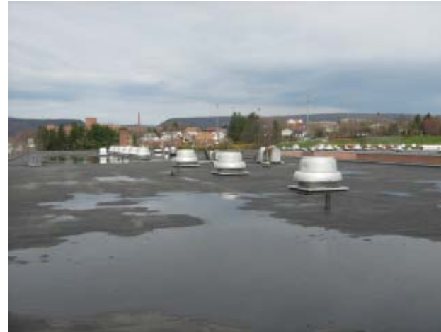
Photo 27 AHS - Roof - fair condition, ponding.
