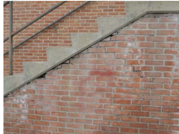
Photo 4 WMS - Masonry – efflorescing, point up required
