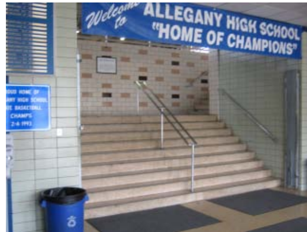
Photo 36 AHS – Non-code compliant stair, high risers
