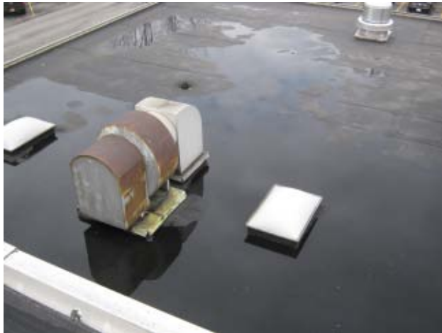
Photo 2- WMS - Roof-condition, fair with ponding
