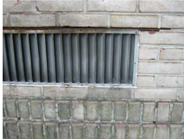
Photo 19 BMS - Exterior rusting lintels
